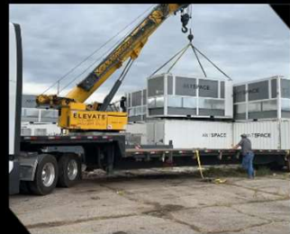
Mining Site Construction
